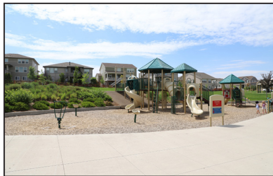
This playground is located on the fringe of a regional detention pond, and can withstand inundation by stormwater runoff. A rubber mat is recommended in lieu of bark or rock to minimize maintenance costs during flood events and to provide a safe surface for children.
