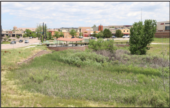
This regional detention pond is located in a public plaza, providing visitors views of a natural green space in an otherwise urban environment.
