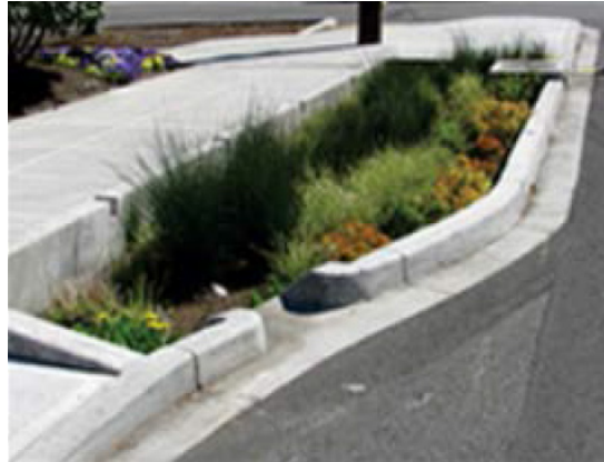
Example of plantings in a bioretention area along rights-of-way.
