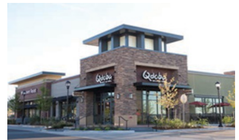
The placement and design of this building promotes pedestrian activity.
