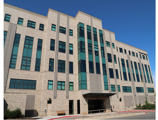
Vertical window patterns relate to the look of this traditional architecture.
