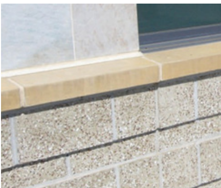
Small changes in planes and materials can create effective shadowing.
