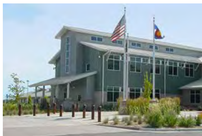
Public Works Facility example
