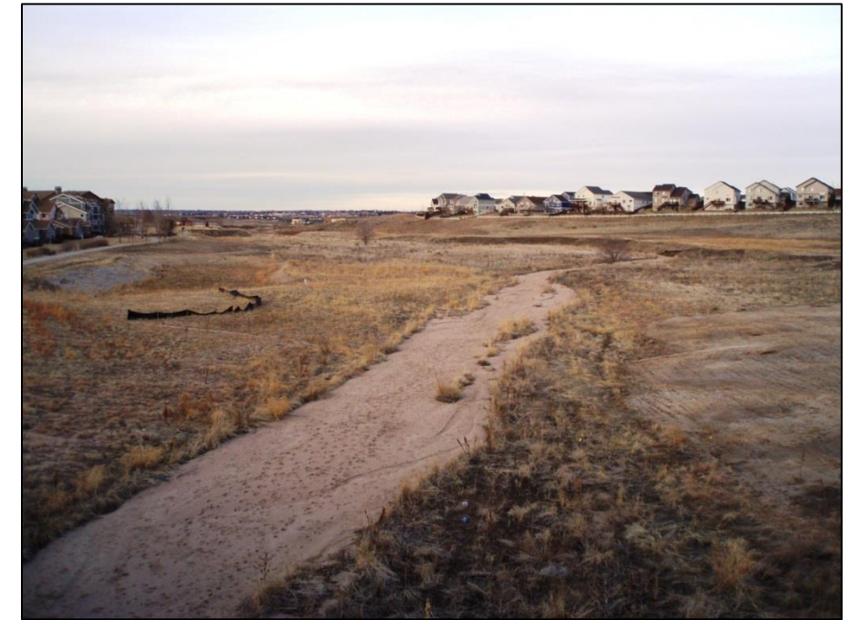
Figure 4-3 - Reach 8 – Town of Parker Sparse, bunchy vegetation with sandy, aggraded low-flow Mid-Range Manning's 'n': 0.03 (overbank) / 0.03 (channel) High-Range Manning's 'n': 0.04 (overbank) / 0.035 (channel)
