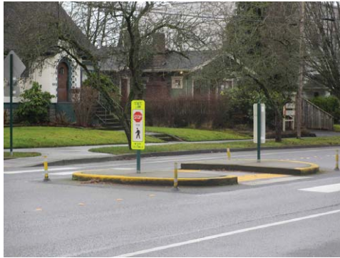
Median Refuge Island
