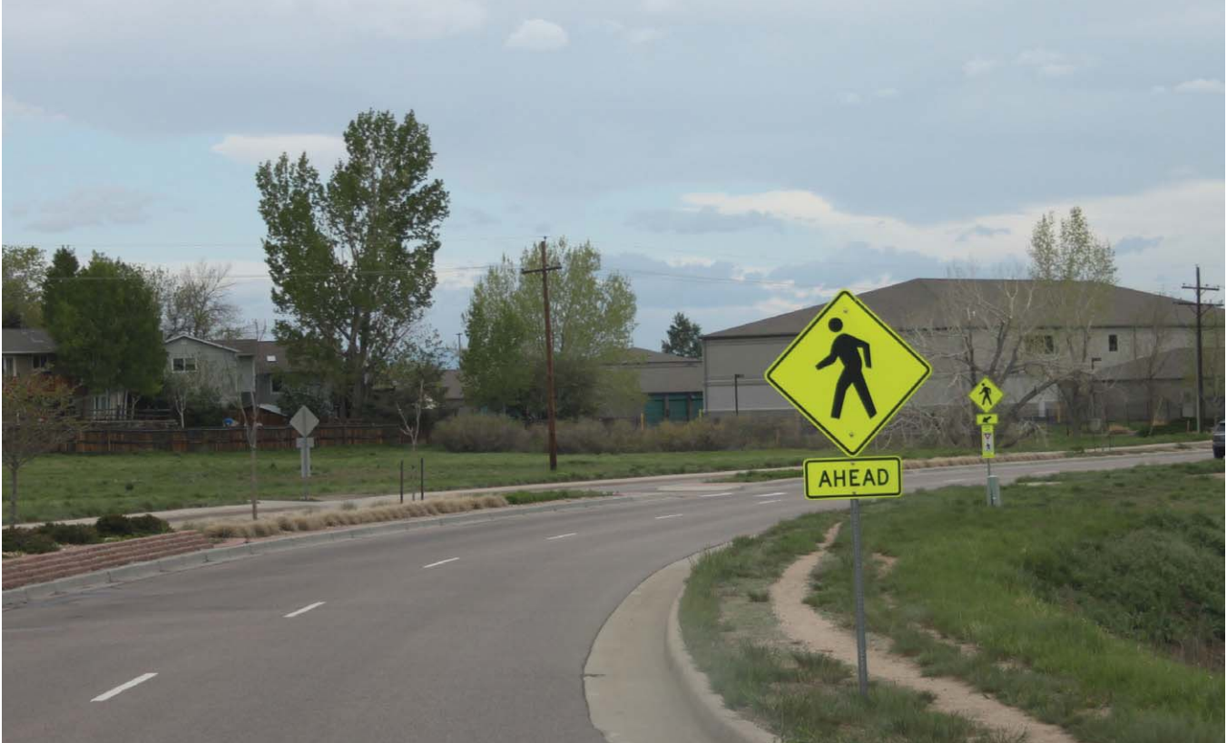
With no sidewalk present, pedestrians walk alongside this residential road as indicated by the social path on the right side of the picture.
