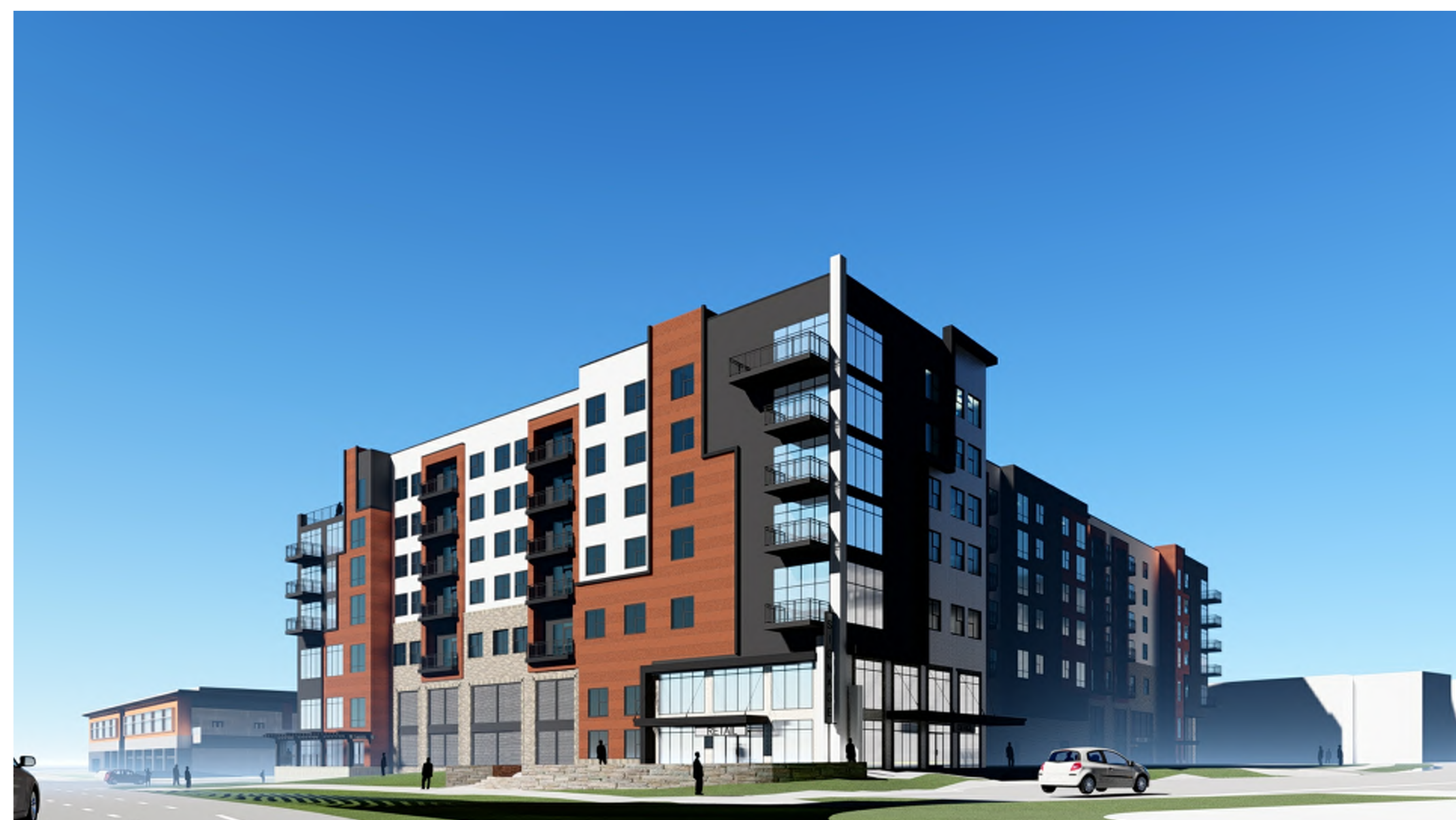
SOUTH EAST CORNER
