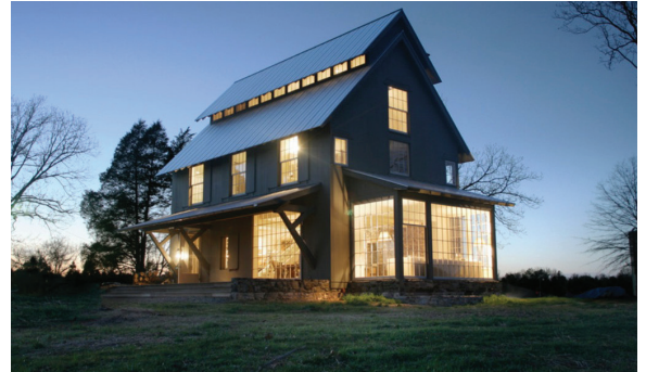
Example of multi-purpose and gathering space architectural forms
