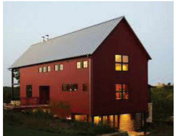
Example of multi-purpose and gathering space architectural forms
