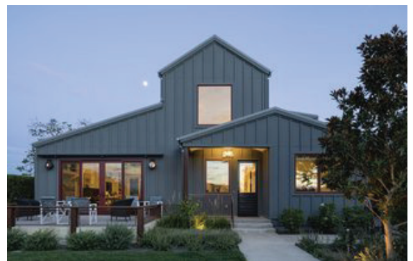
Example of multi-purpose and gathering space architectural forms
