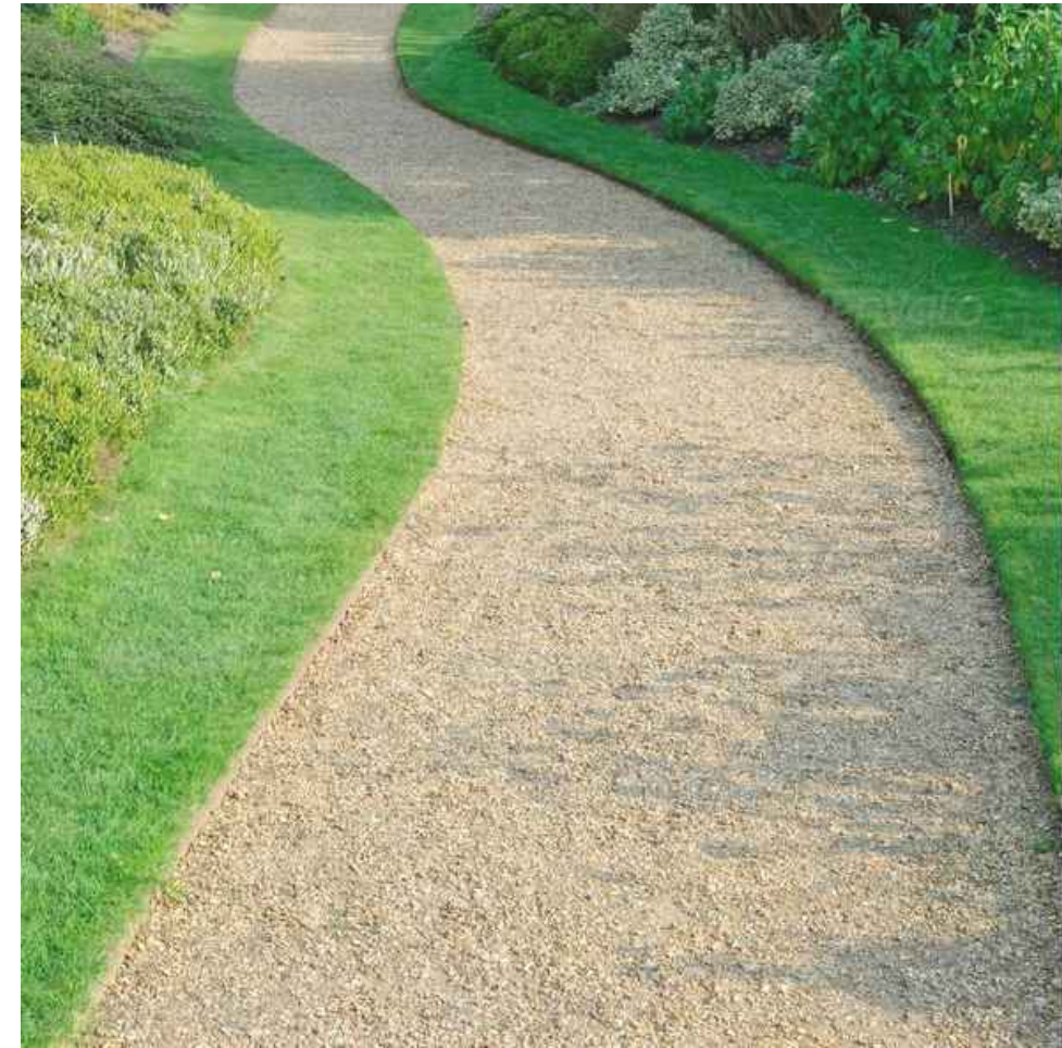
SOFT SURFACE PATH TAN CRUSHER FINES, 4" DEPTH, APPROXIMATELY 5' WIDTH.
