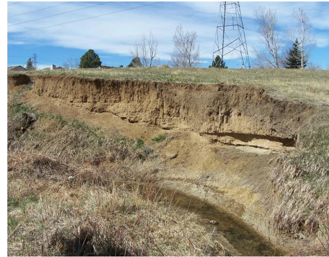
FIGURE 4-3 Channel bank erosion, Greenwood Gulch
