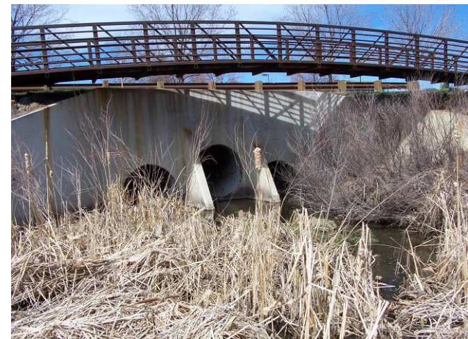
FIGURE 4-1 Quebec Street crossing on Greenwood Gulch
