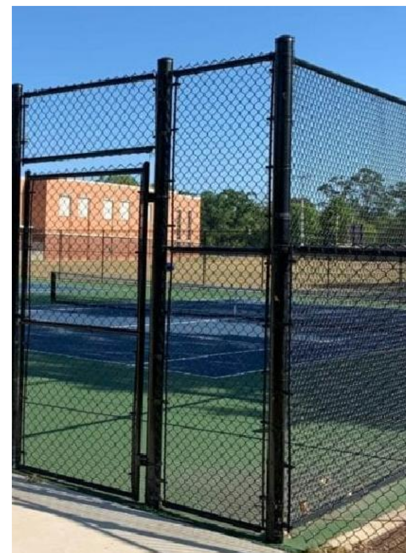
COURT CHAIN LINK FENCE (H) CHAIN LINK / BLACK COLOR COAT
