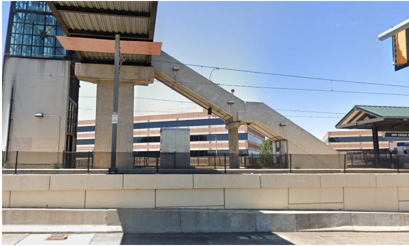
DRY CREEK RTD STATION
