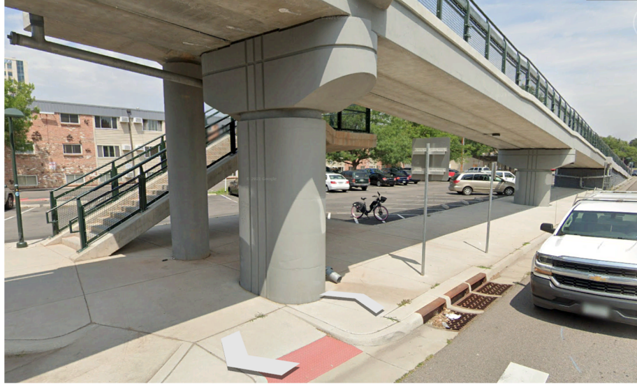
COLORADO CENTER BRIDGE
