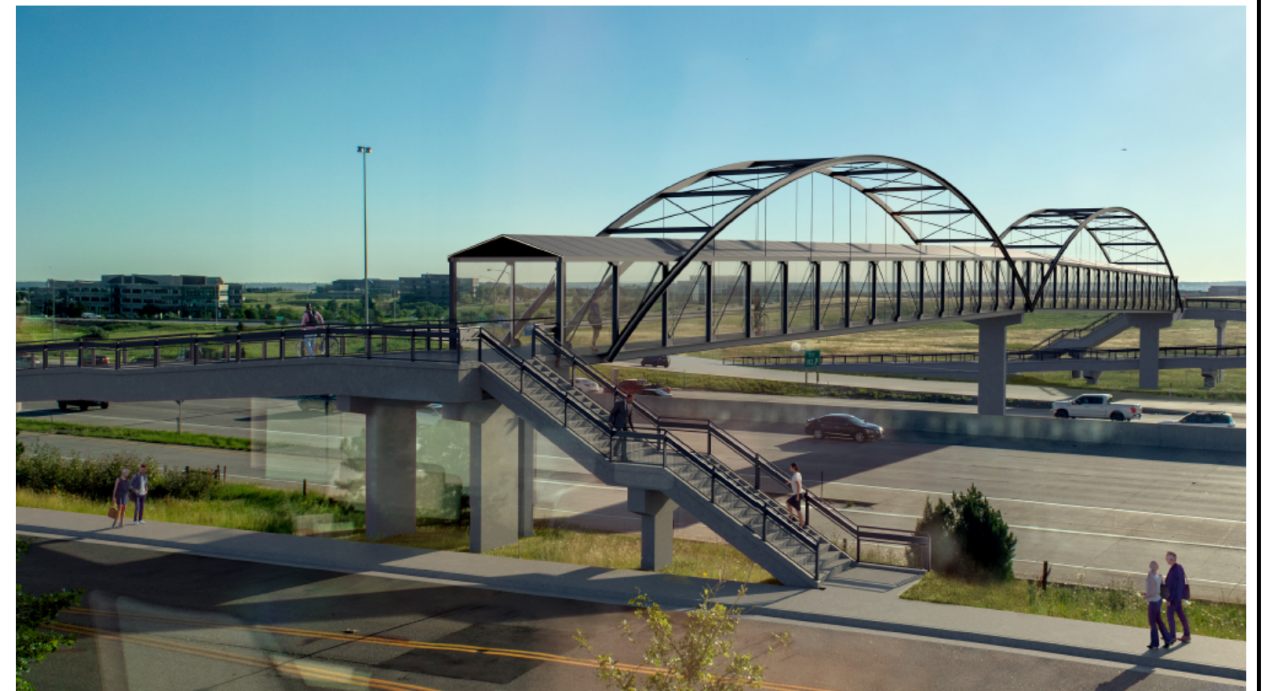
VIEW OF PEDESTRIAN BRIDGE FACING NORTHEAST
