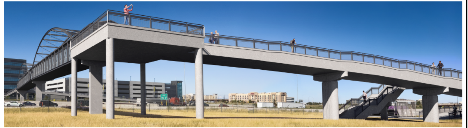
VIEW OF PEDESTRIAN BRIDGE FACING NORTHWEST
