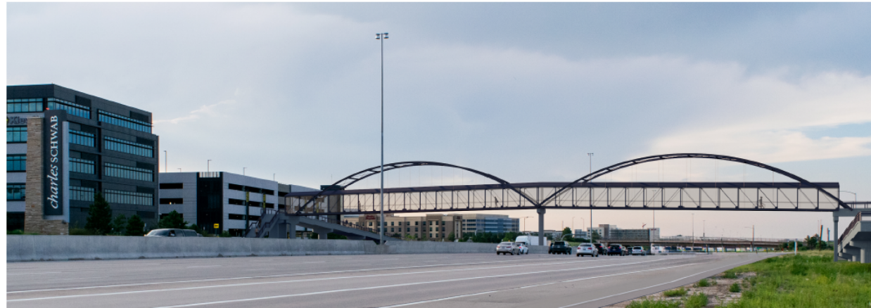
VIEW OF PEDESTRIAN BRIDGE ON NORTHBOUND I-25
