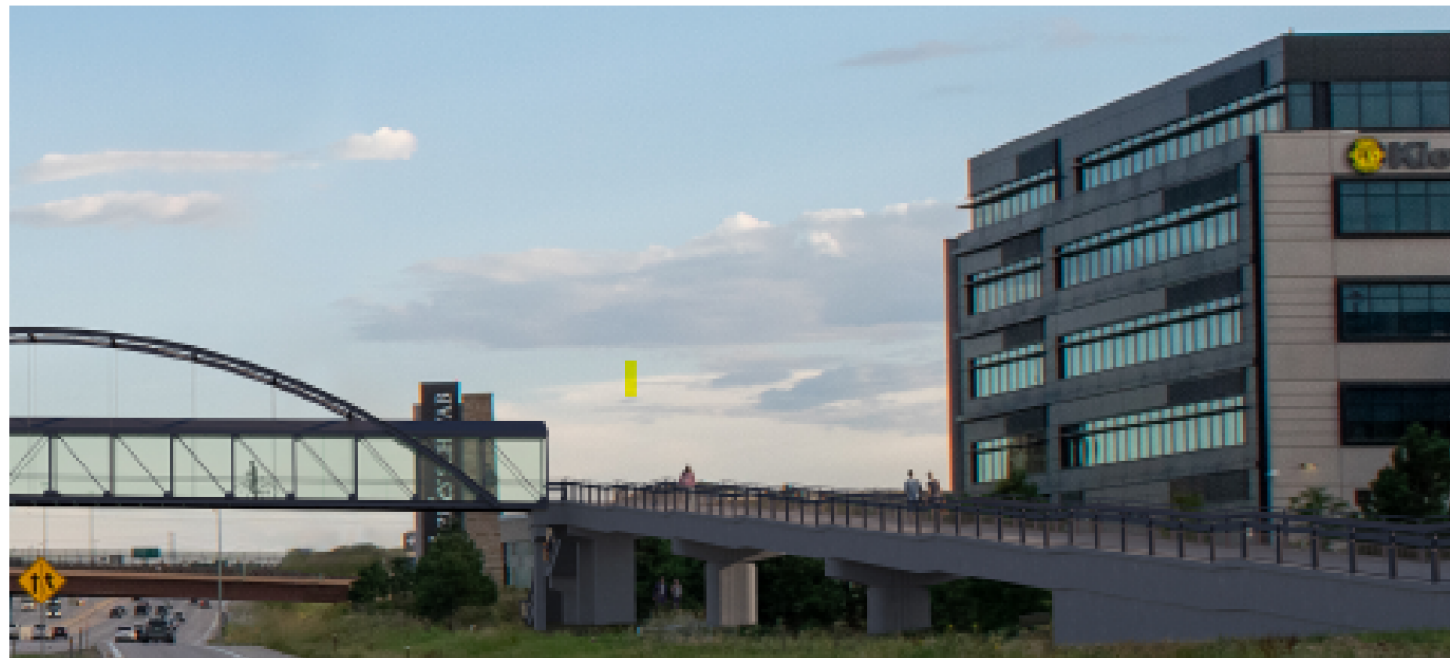
VIEW OF PEDESTRIAN BRIDGE FACING SOUTHWEST
