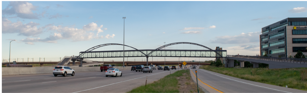
VIEW OF PEDESTRIAN BRIDGE ON SOUTHBOUND I-25
