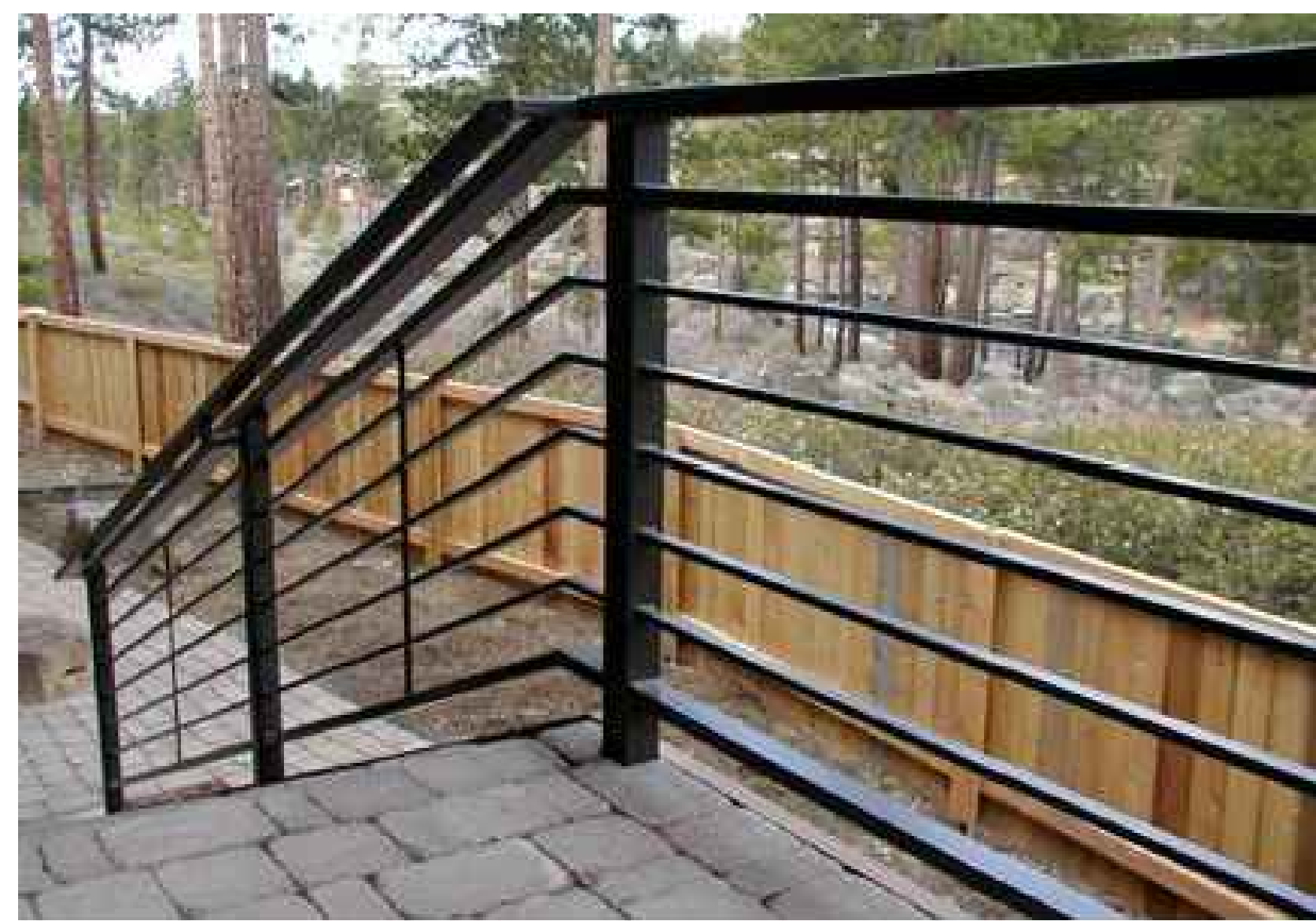
METAL HAND RAIL TO BE CUSTOM FABRICATED ON SITE. HEIGHT 36", COLOR BLACK
