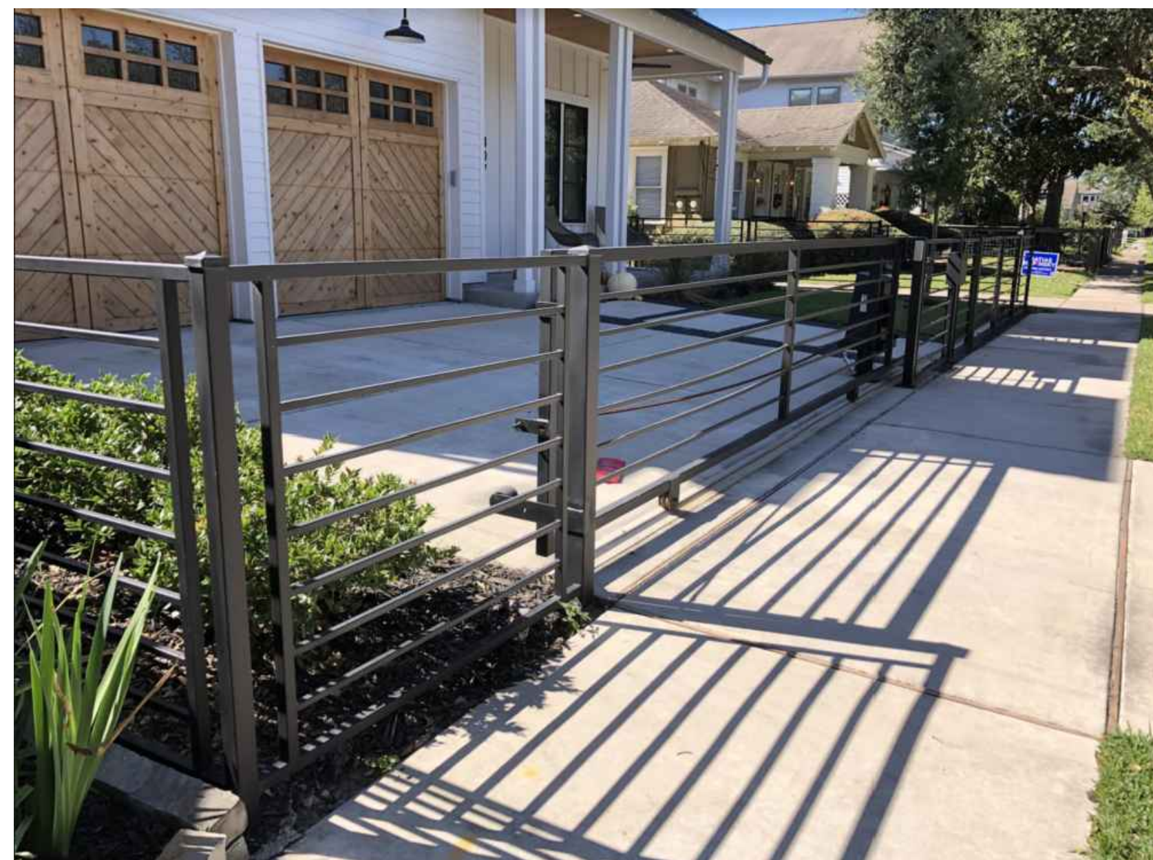
METAL FENCE TO BE CUSTOM FABRICATED ON SITE. HEIGHT 36", COLOR BLACK
