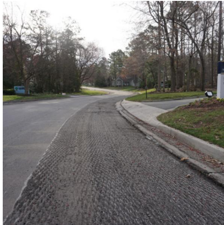
Detail Mill & Overlay
