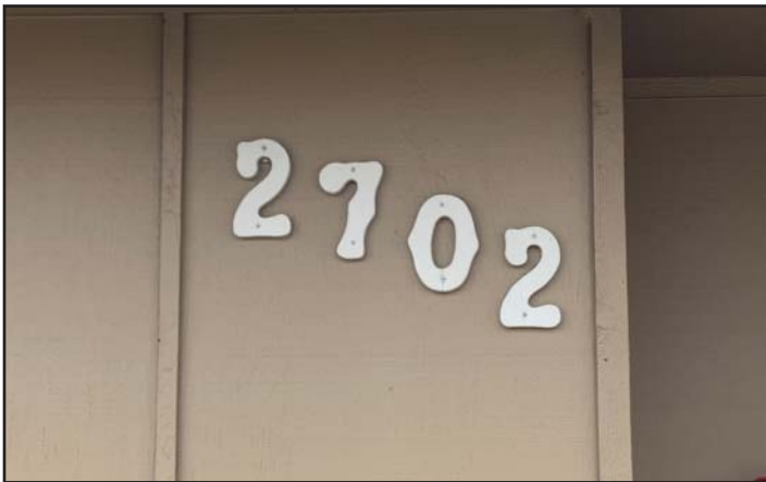
This address is posted effectively. Photo by South Metro Fire Rescue.
