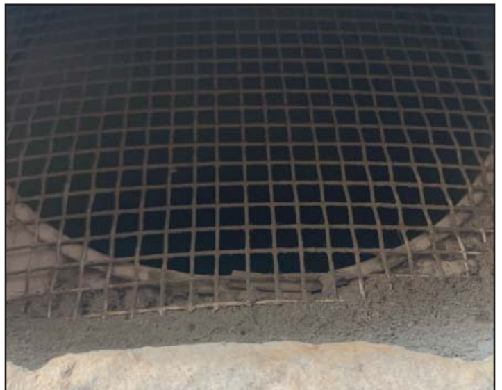
All vents should have screening with holes no bigger than 1/8 of an inch to reduce the likelihood of viable embers from entering a structure. The vents at right are protectect properly. Photos by South Metro Fire Rescue.
