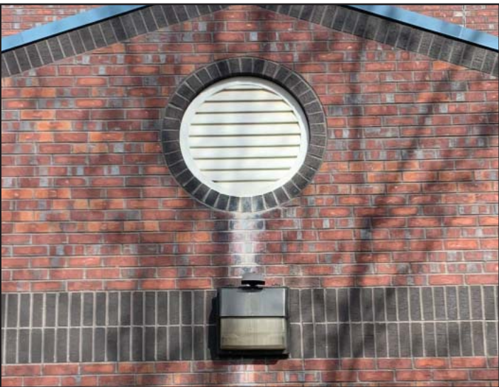
There are several different types of vents commonly used for attics. The two upper images are soffit vents. The photograph below shows a gable vent. Photos by South Metro Fire Rescue.
