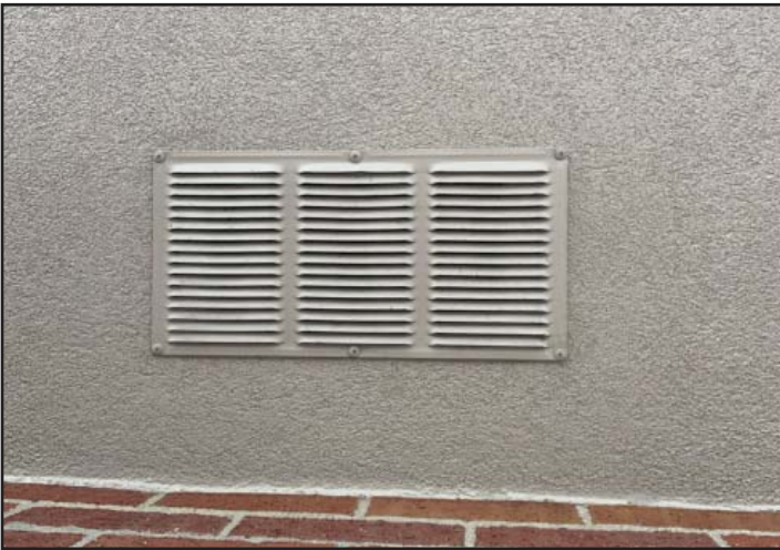
There are several different types of vents commonly used for attics. The two upper images are soffit vents. The photograph below shows a gable vent. Photos by South Metro Fire Rescue.
