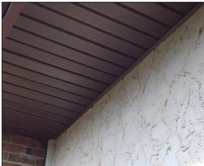
The eaves in the images above and below are protected by fire-resistant soffits. Photos by South Metro Fire Rescue.
