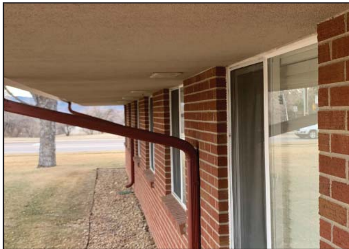
The eaves in the images above and below are protected by fire-resistant soffits. Photos by South Metro Fire Rescue.
