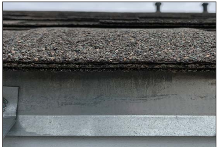
This image shows a drip edge, which helps protect the roof assembly from moisture and embers. Photo by South Metro Fire Rescue.
