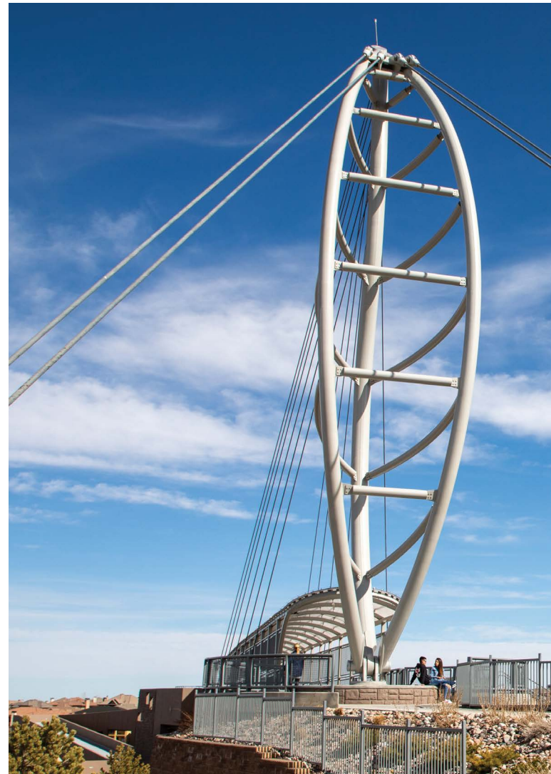
Photo taken in 2020 - Lincoln Avenue Pedestrian Bridge
