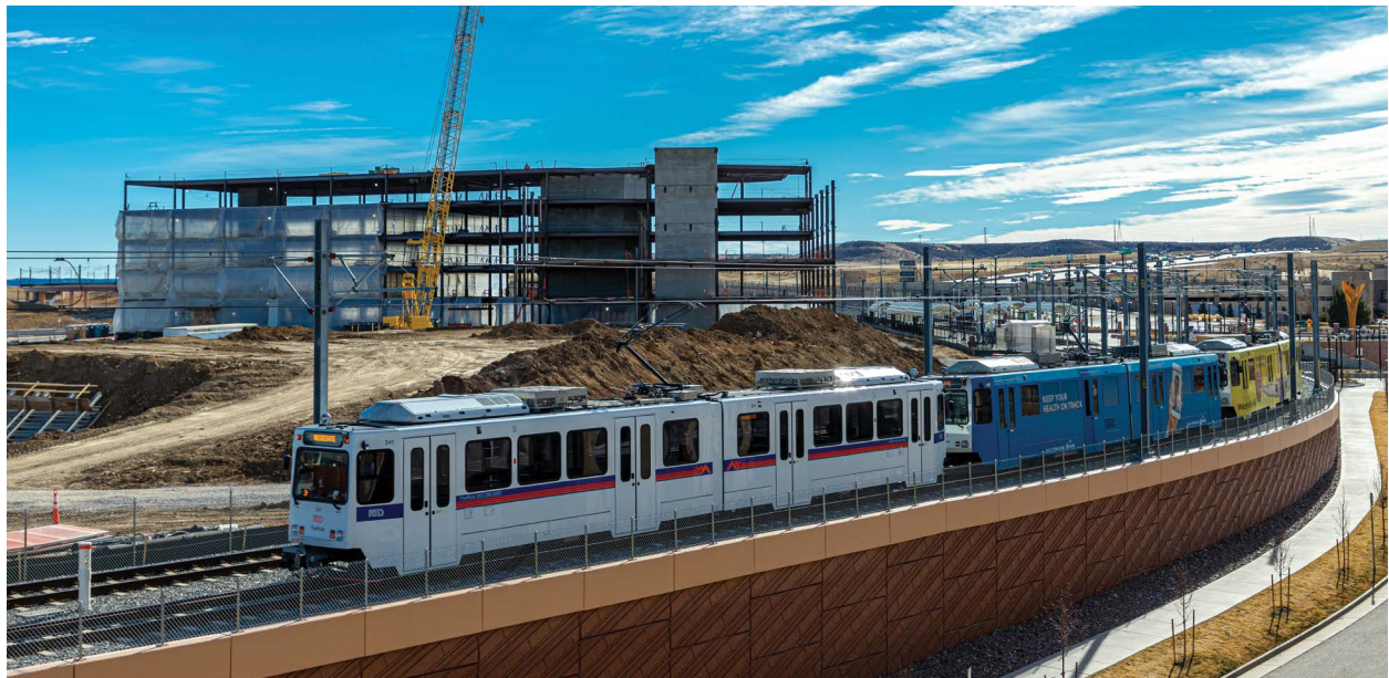
Photo taken in 2020 - Kiewit construction site
