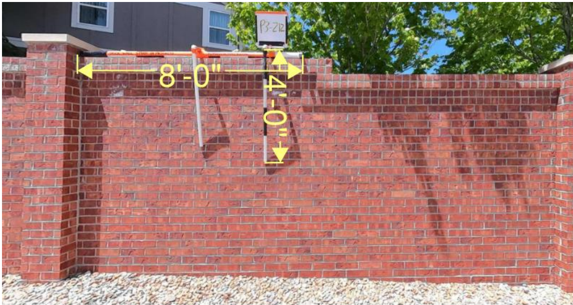
Figure 14. Rectified and scaled photograph of panel P3-212, showing 8'-0" long horizontal story pole and 4'-0" tall whiteboard pole.
