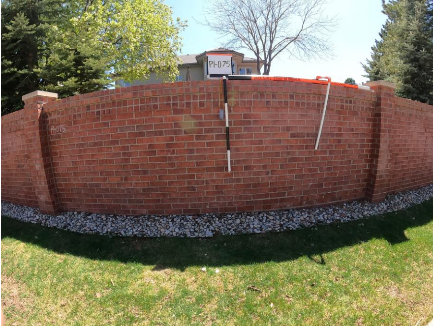
Figure 12. Unrectified photograph of panel P1-075.
