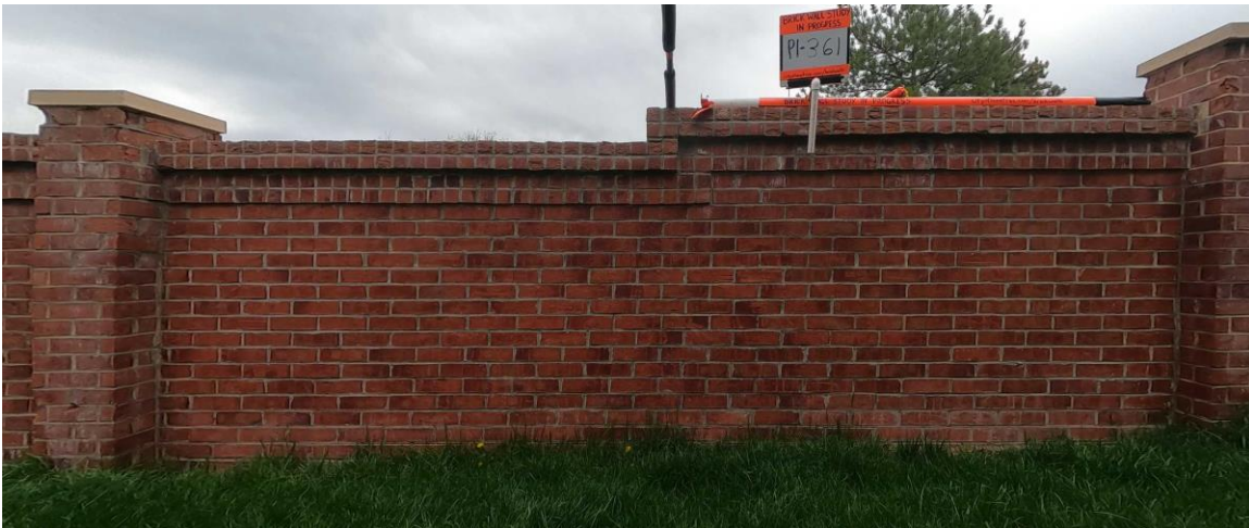
Figure 9. Typical panel photograph from the yard side.
