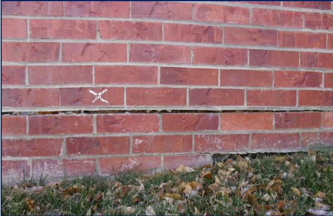
Figure 67. Sagging at P1-323 as photographed in 2011.
