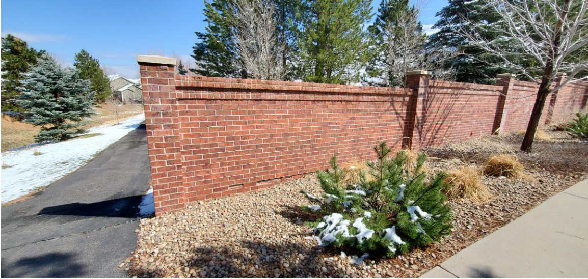
Figure 1. Overall view of typical brick wall panels.
