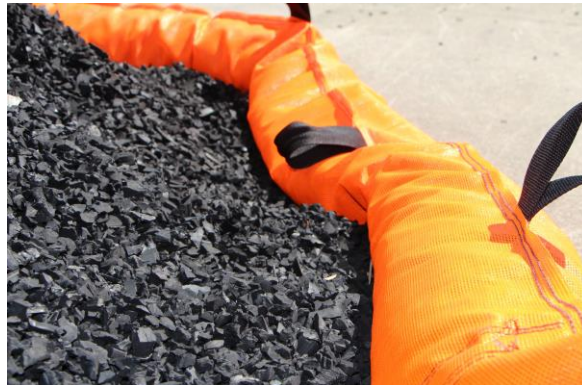
Protect downstream side of stockpile
