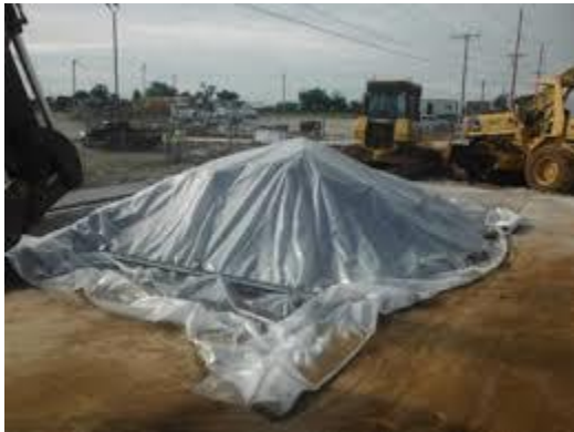
Cover stockpiles when not in use
