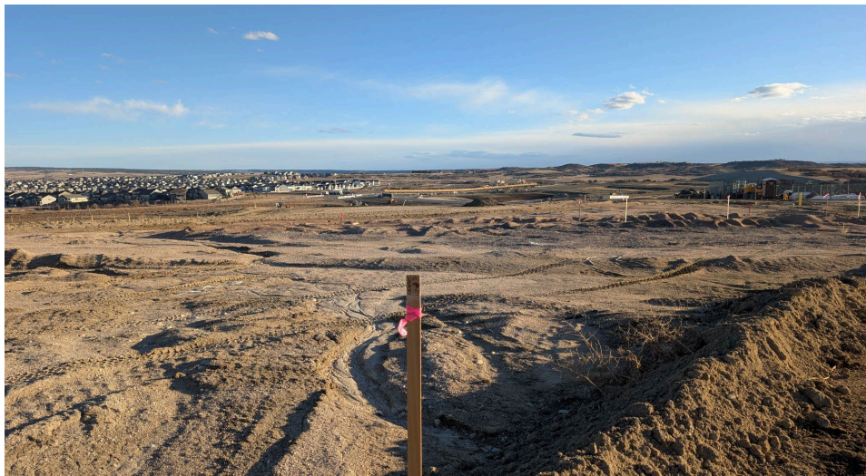
Photo No. 6 Location: Boring B-13 Site development is ongoing at the Rueter-Hess site and along Stroh Road.
