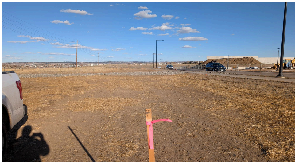
Photo No. 4 Location: Boring B-7 View of Boring B-7 and North Ridgeway Parkway.
