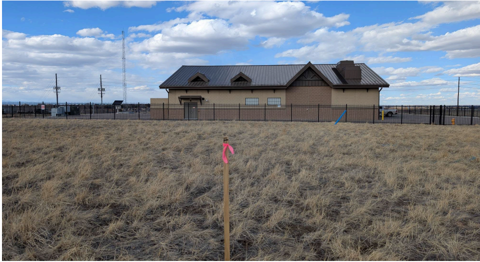
Photo No. 5 Location: Boring B-11 Existing Ridgeway Well House.
