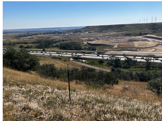
Description: View of I-25 wildlife underpass from Property View Direction: East
