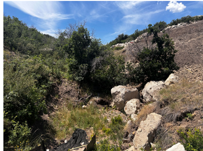
Description: Drainage area leading to culvert View Direction: South
