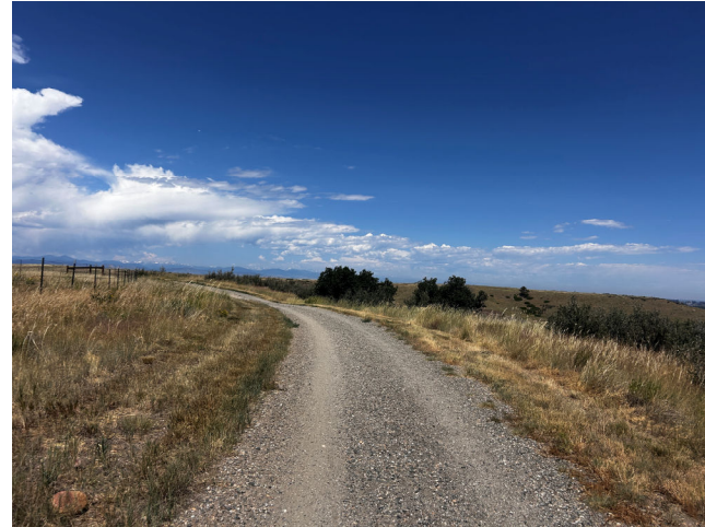
Description: Access road along ridge View Direction: West
